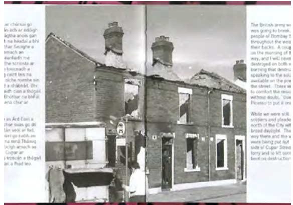
Fig. 12 Image showing the destruction of Bombay Street after the houses were burnt to the ground Image copyright Ciaran Mackel's archive
