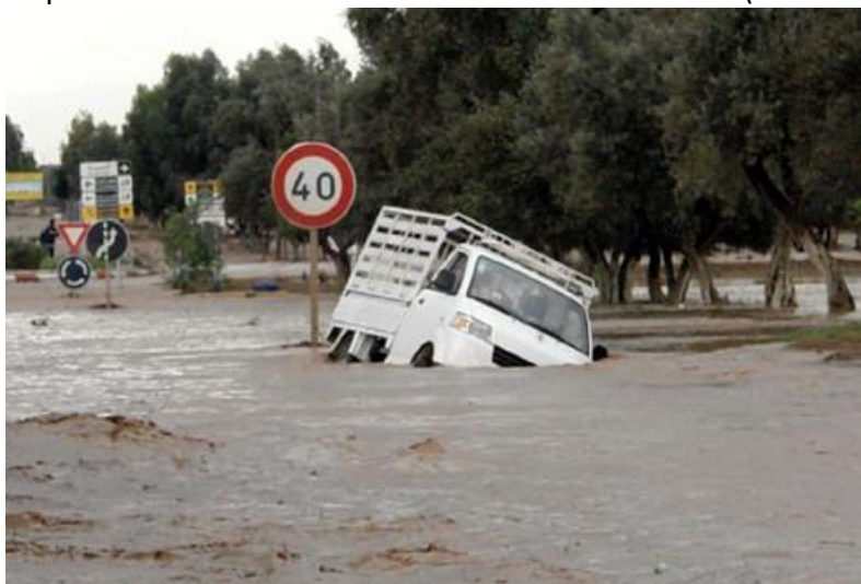
Figure 4. Impacts of floods on roads infrastructures in Nador (November 2008).
